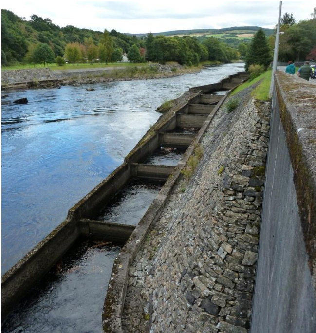
Pitlochry dam fish passage ladder
